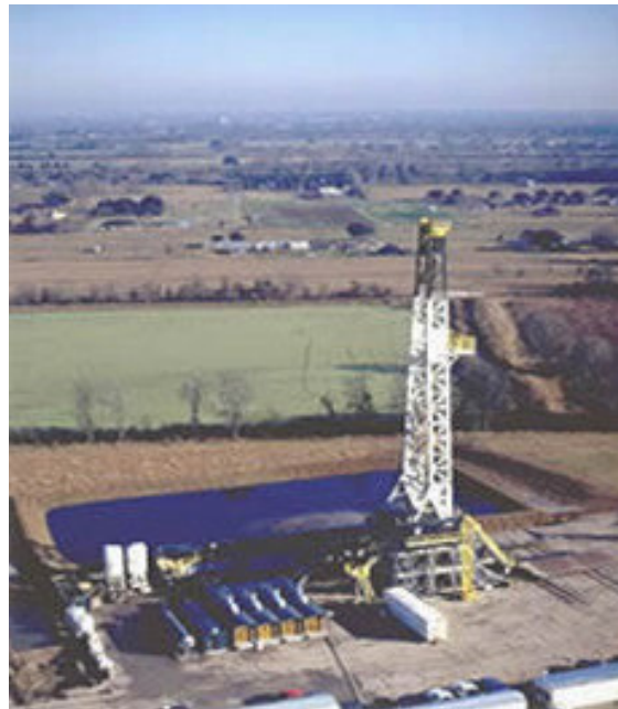
Grey Wolf drilling rig
