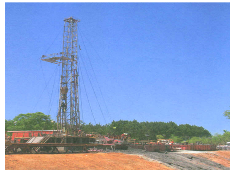
Spencer Harris 7000 rig to be used
